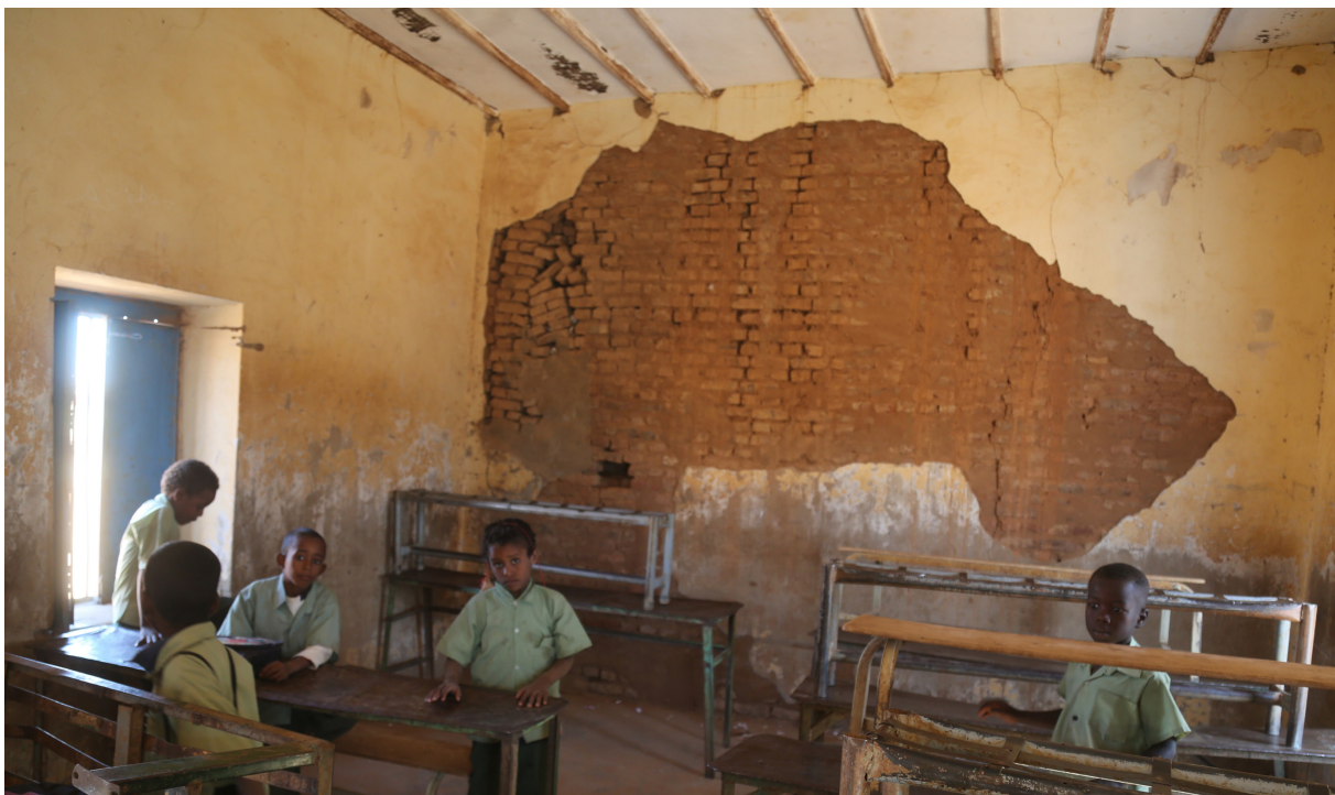
Learners in one of the classrooms at a flood affected school in Wad Soba. The level and effect of flood water is still visible on the walls.
