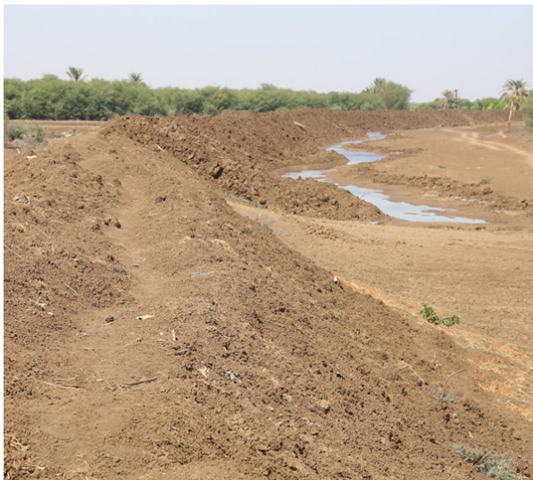
A clear view of heaped gravel contour barriers erected around Wad Ramli to block floods
